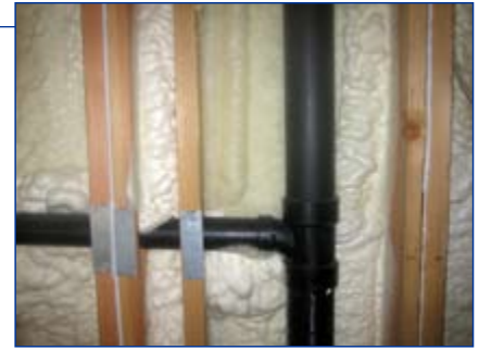
Spray foam insulation installed by JB Insulation of Sherwood is up to 40% more efficient than traditional fiberglass
